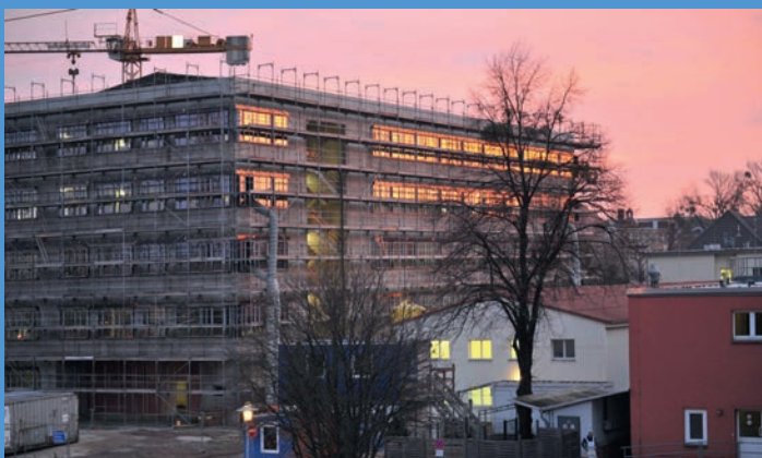
DZNE in der Bauphase The DZNE during construction
